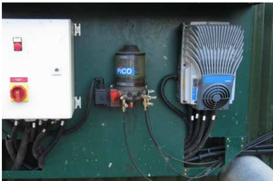
VACON® 100 X installed outdoors. To turn the paddle agitator and ensure optimal operation, a VACON® 100 X AC drive and an automatic central lubrication unit are used.
