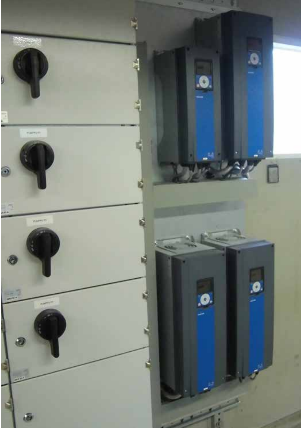
VACON® 100 FLOW units at the Osvald waste water pumping station. The drives were installed on a backplate at SK-kojeisto, the Seinäjoki, Finland based company that has built the switchboards used at KRS-Vesi.
