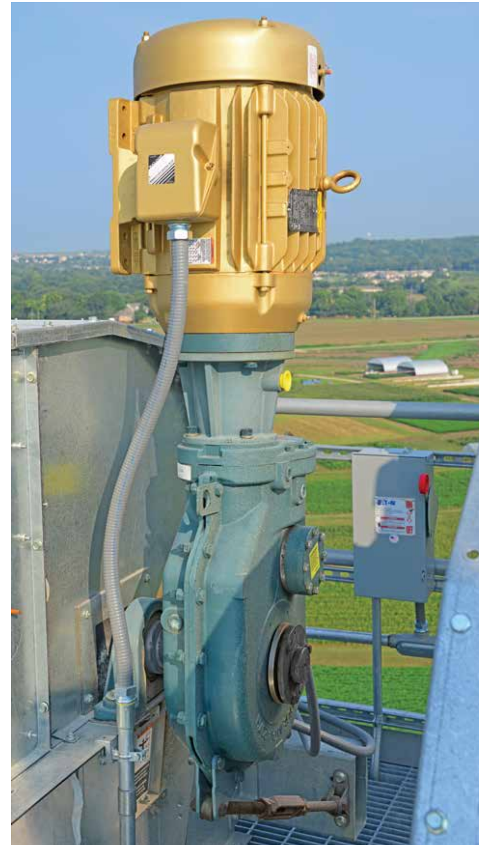
For the bucket elevators, SCAFCO chose Baldor's Dodge Motorized Torque-Arm II® (MTA) gear reducers, a heavy-duty, right-angle beltless Torque-Arm, for its ease of maintenance and its compact, space-saving design. It also selected Baldor•Reliance® Super-E® premium efficient motors, which run cooler and longer with better reliability than any other industrial motor.
