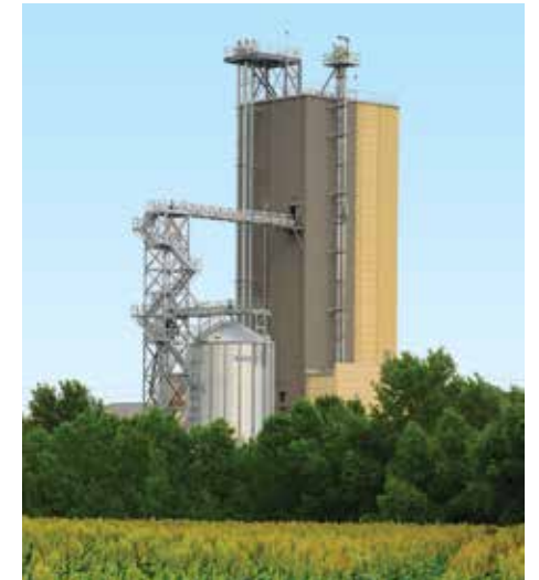
ASI-Industrial, the subcontractor responsible for building the slip-formed concrete main tower, also approved and installed all the equipment in the facility. ASI specified Baldor products almost exclusively on its projects and was not surprised that other OEMs participating were also choosing Baldor.
