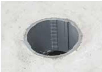
Cut box top level with concrete
