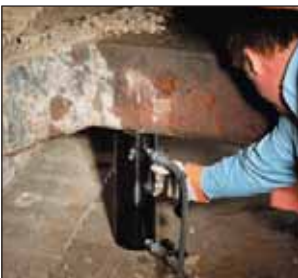
◀ An RAR-506 was easy to position under a bulldozer for repair of frame member.
